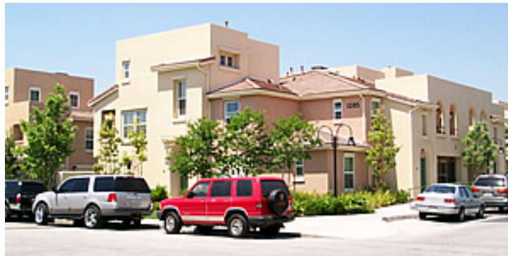
Figure 13: Another example of a community with a 20 du/ac density shows each individual family dwelling with yard space and driveways. (Building Healthy Communities 101 What Does Density Look Like in my Neighborhood?)
