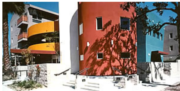
Figure 14: This community has a density of 40 du/ac. Though homes are closer together, a mixed use zoning code is implemented to allow for many amenities within walking distance. Additionally, a highly modern design is introduced to provide a higher aesthetic quality within a community living space. (Building Healthy Communities 101 What Does Density Look Like in my Neighborhood?)
